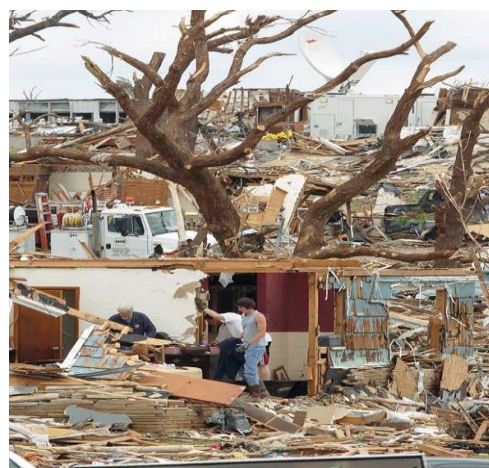
Figure 3: Picture of Destruction from Extreme Weather and Compound Disaster (Grimley et al., 2024).
